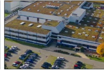
IQAir AG Technology Center Steinach, Switzerland
